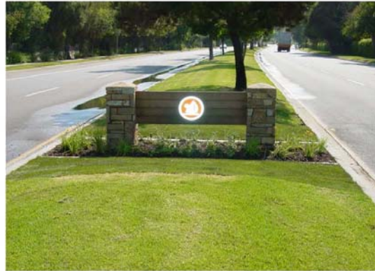
Figure 1: Before Photo with concave design and no infiltration.
